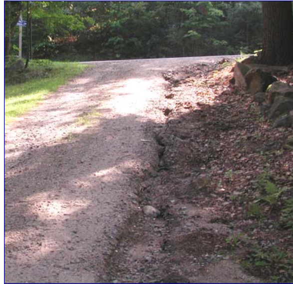
Good ditches are essential to collect road run-off. Above, the ditch has badly eroded, but below (shown from opposite angle), it's been armored against erosion with crushed stone.
