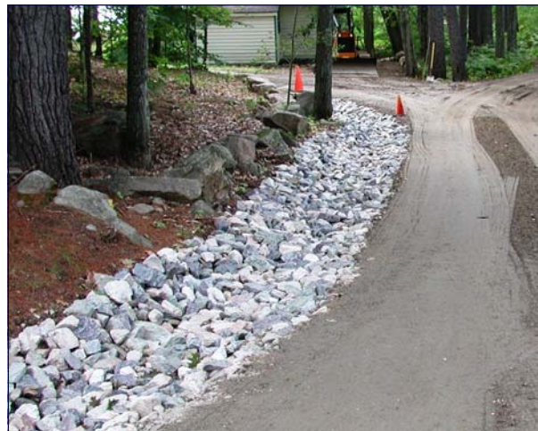
Good ditches are essential to collect road run-off. Above, the ditch has badly eroded, but below (shown from opposite angle), it's been armored against erosion with crushed stone.
